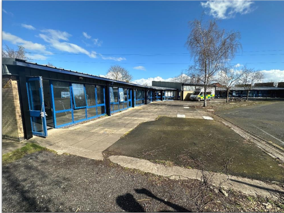
Figure 4.6: A view of the back of the Sheila Scott building. The picture shows many open doors and windows.
