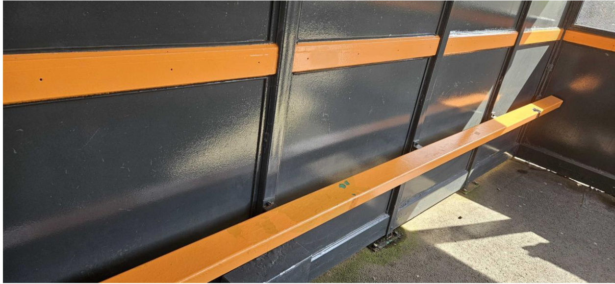
Figure 20: Waiting area seating at Hartlebury
